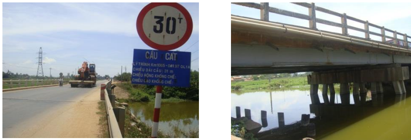
Figure 3: Images of Cat bridge surveyed on June 2011
