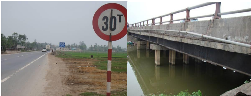
Figure 1: Images of Cua bridge surveyed in January 2011
